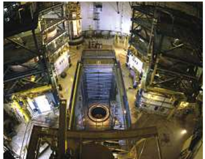
Cattenom, France (4 x 1,300 MWe): inside a reactor building.
